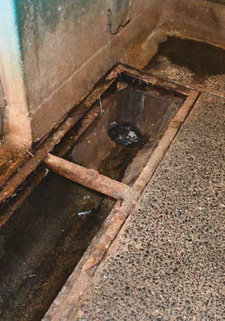
Open drainage along the ward (Kakamega.)
